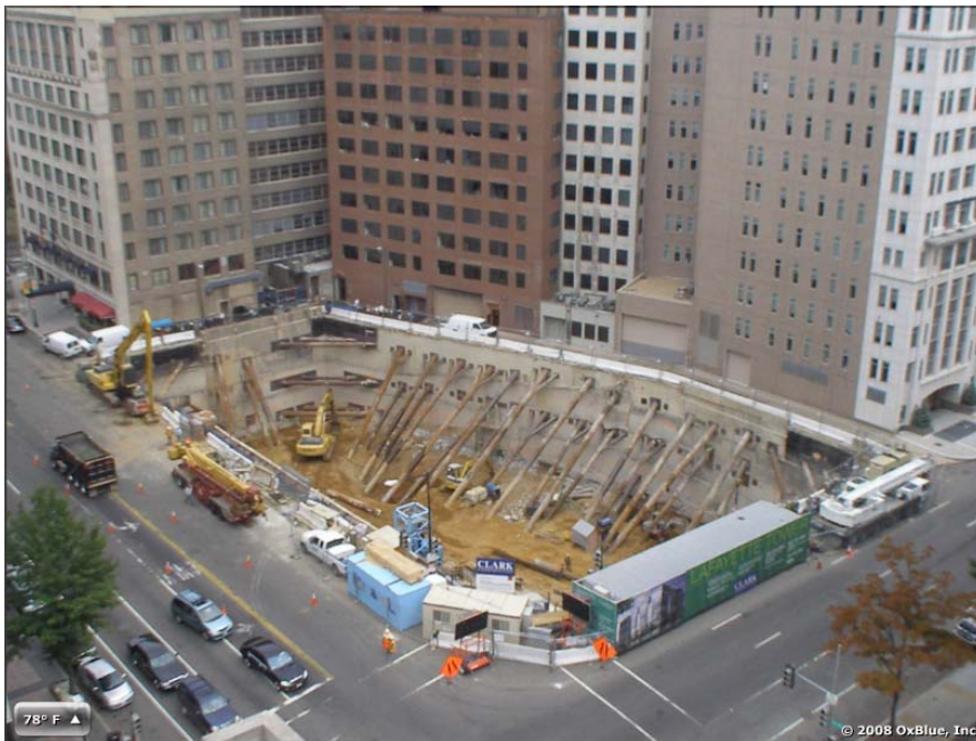
Figure 1 - Demolition Site Picture
