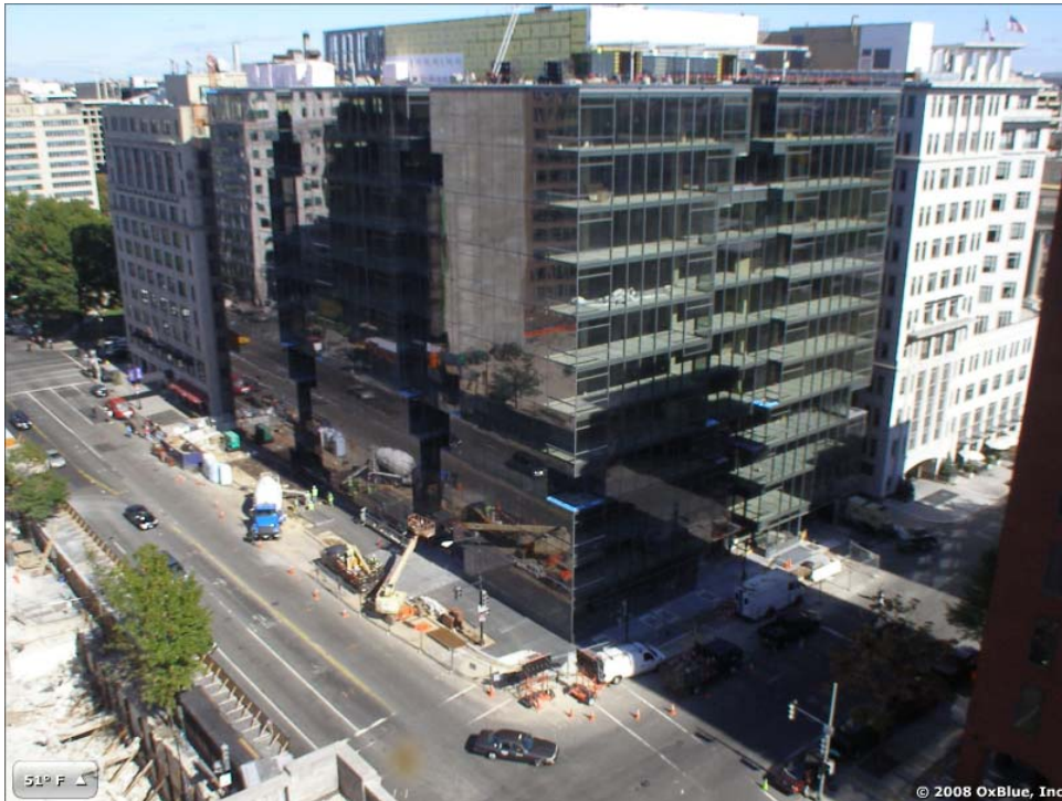
Figure 3 - Finishes Site Picture
