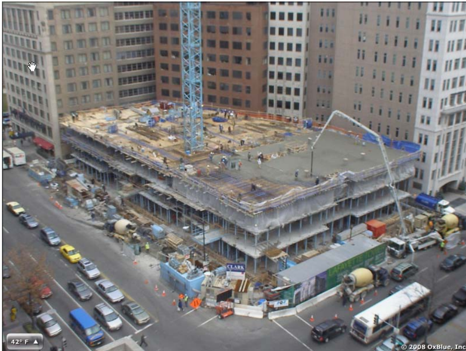
Figure 2 - Superstructure Site Picture
